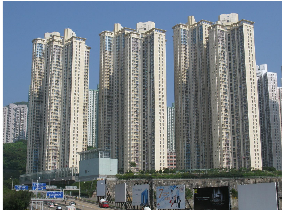
Harmony Block (1990s) – Yau Lai Estate 40-storey
