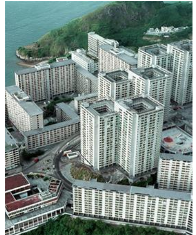
Twin Tower (1970s) Wah Fu Estate 20-storey
